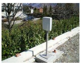
Microwave barrier are generally used between the external perimeter and inner perimeter and on detection it sends a visual alarm in the zone associated with audio alarm in the control panel. As the frequency is very high, it is not affected by wide range environmental conditions and thus false alarm rate is very low.
